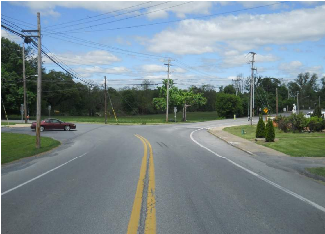
Direction / Road: WB Cornwall Road/Boyd Street Approach / Departure: Approach Distance: 50 Feet
