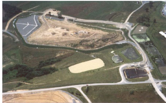
Aerial Photo of GLRA Landfill
