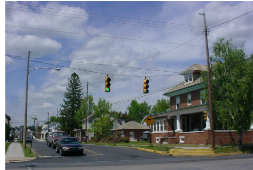
Stairs in NE quadrant of Center Street and US 422
